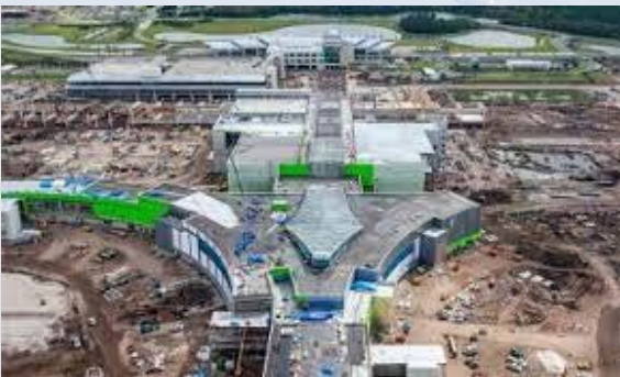
GOAA STC Fiber Backbone and GPON Network Implementation $ 1,500,000.00
