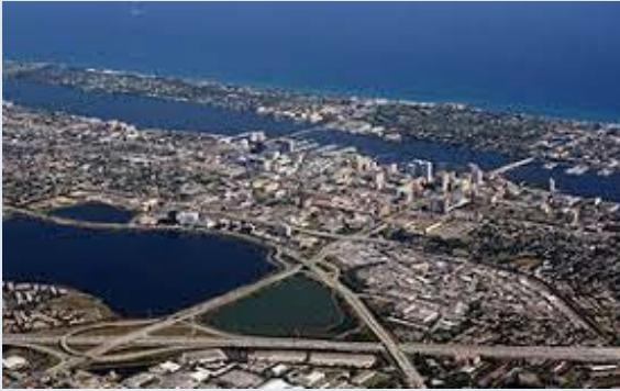
Palm Beach County - County Wide Design - Build Fiber Network $9,600,000
